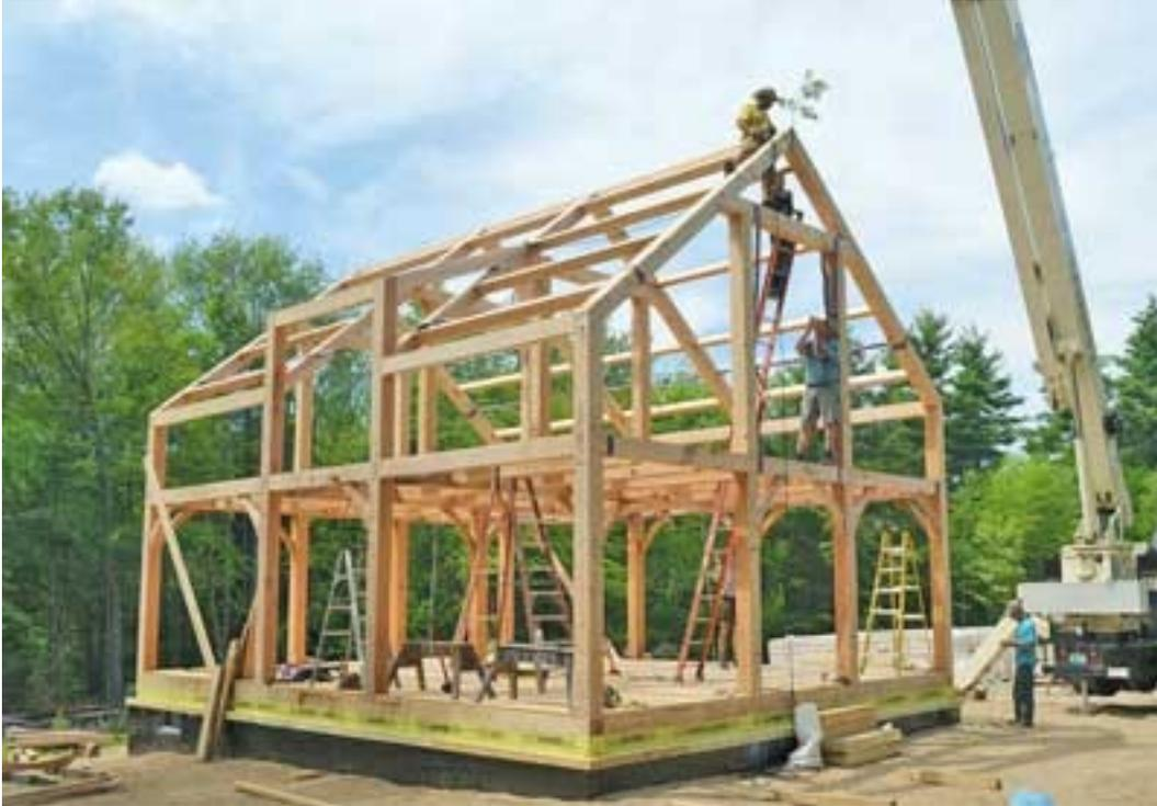
**COMPLETED FRAME — All the beams in the frame were prepared over several weeks, then connected and put into place in a single day. A sprig of pine was affixed to the top of the house in accordance with an old tradition. Photo by Jon Hardie**
